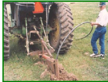
Shallow ploughed installation of pasture pipeline
