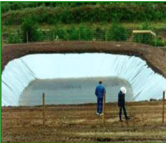
Raised earthen storage with woven polyethylene liner
