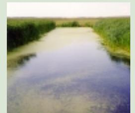
Construction of "deep zones" in the wetland cells is a design feature to help distribute wastewater and prevent short circuiting across the surface of the cell.
