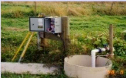
Pump control panel and wetwell containing submersible pump.
